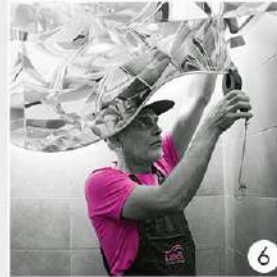
Hanging the ceiling with clips
